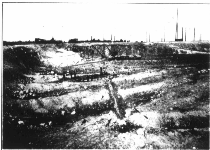
General View, showing Excavation.
