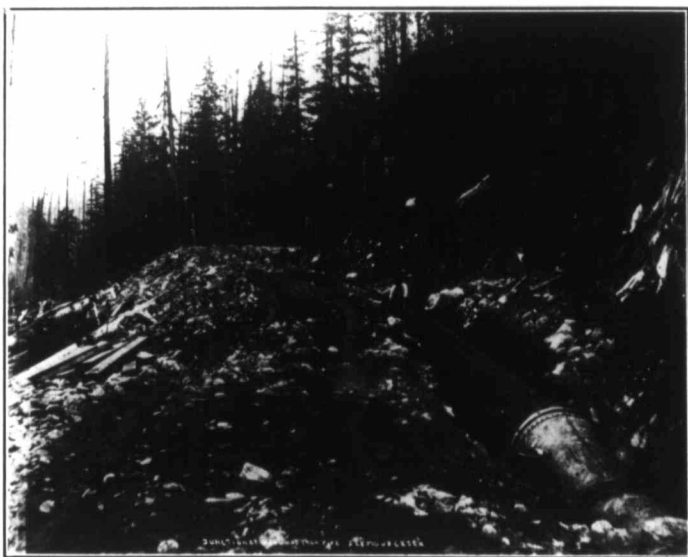
Junction of Wood and Iron Pipe, Seymour Creek.
