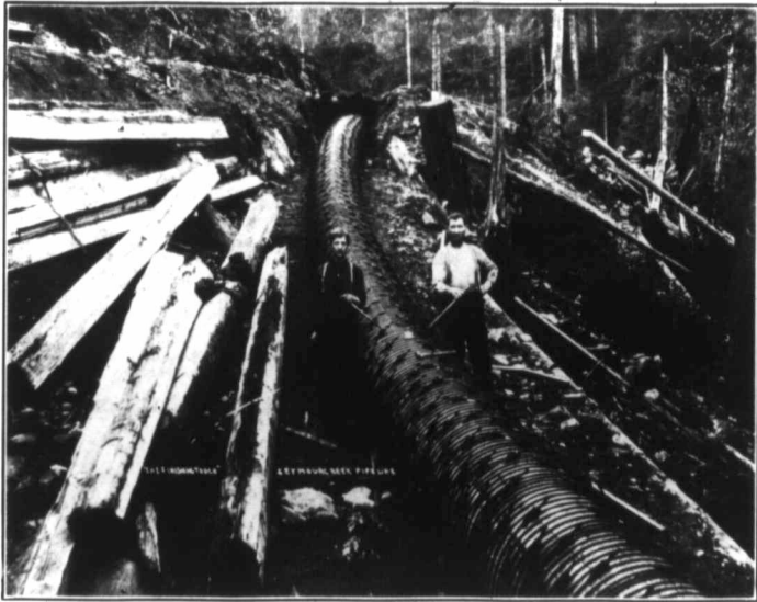
"The Finishing Touch," Seymour Creek Pipe Line.
