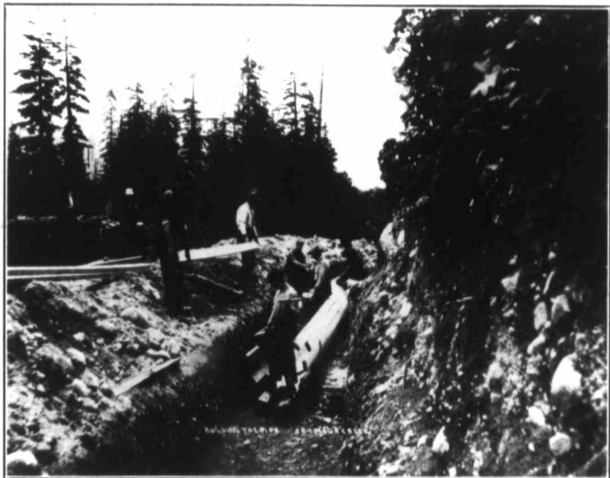
Building the Pipe, Seymour Creek.
