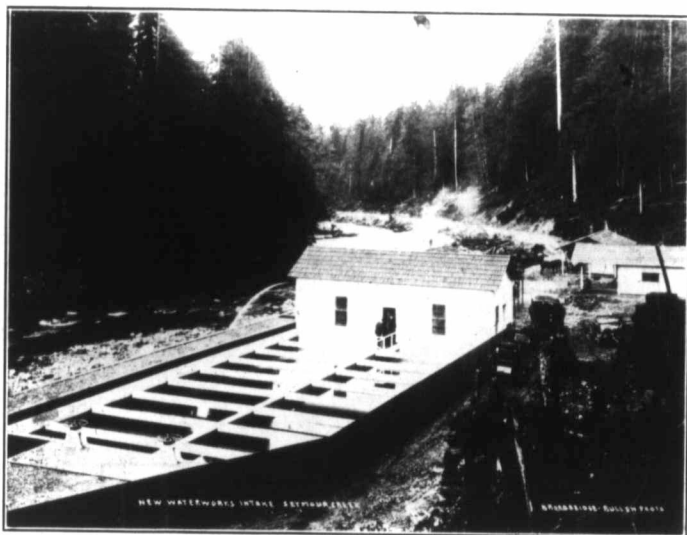
New Waterworks Intake.
