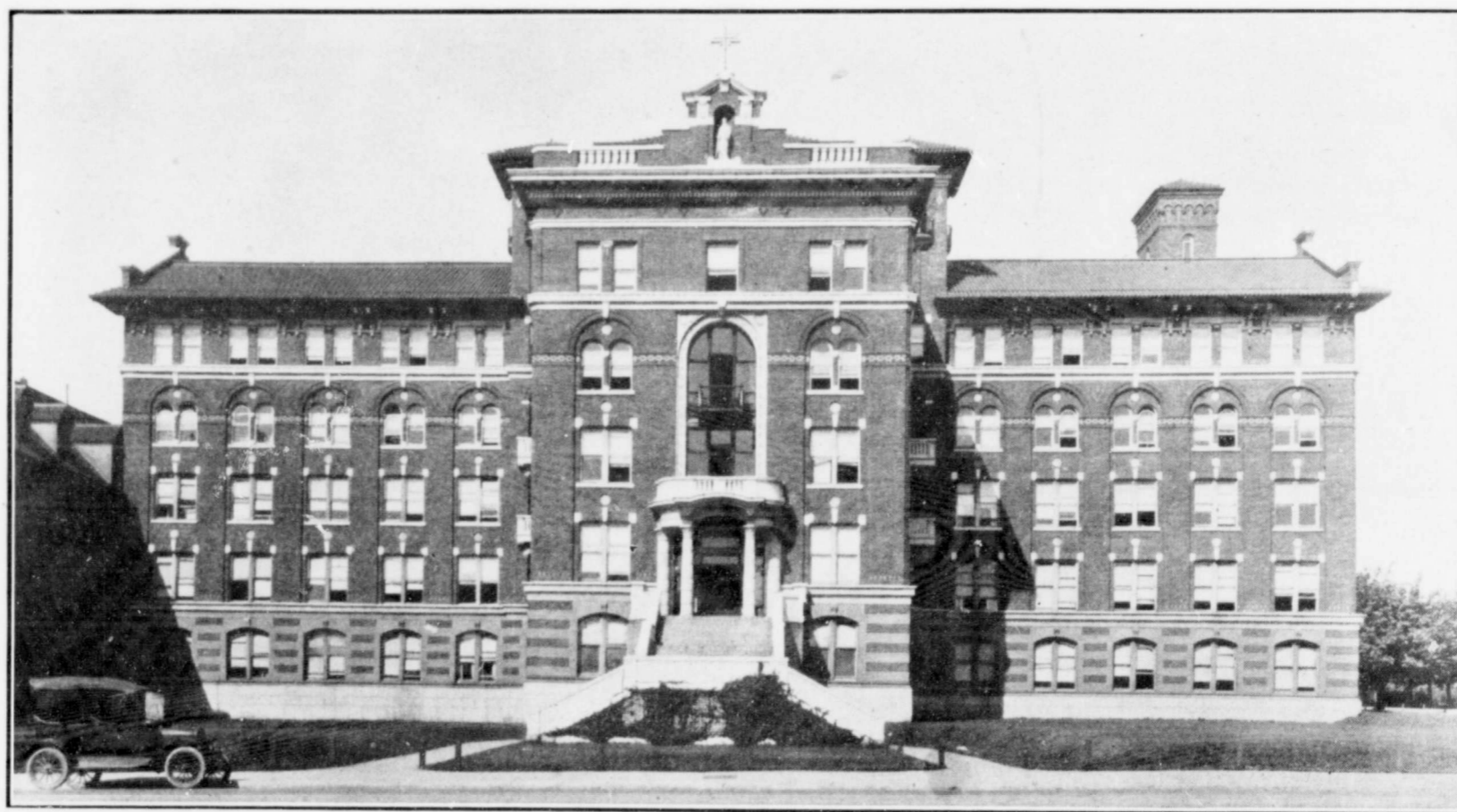
ST. PAUL'S HOSPITAL, VANCOUVER, B. C.
