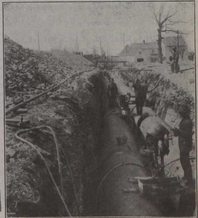
Fig. No. 7.—Riveting Pipe in Trench
