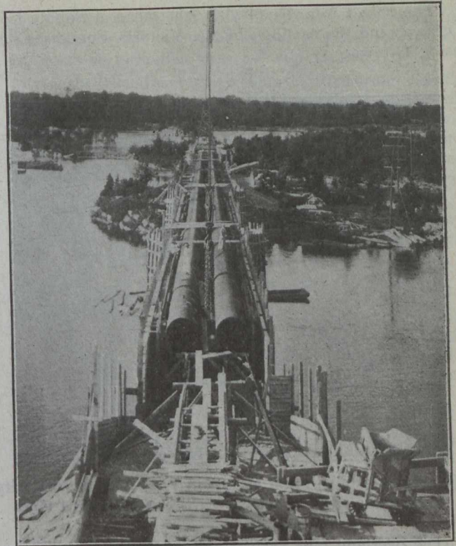
Fig. No. 6.—Twin Pipes Laid Across Lemieux Island Bridge
