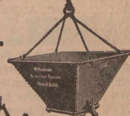
57—Steel Coal Box with Drop Bottom
