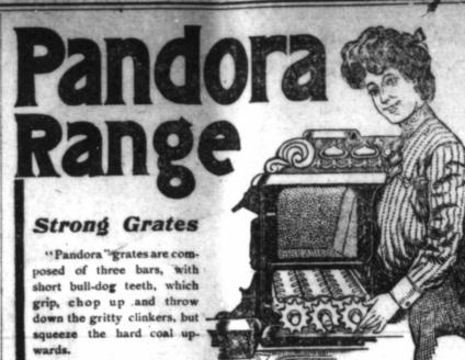
The two outer bars work on the centre one, and all three are held together in one strong iron frame, which can be removed by merely unscrewing one bolt. This is a great point in a range. Most range grates require expensive experts to take out old ones and put in new grates You can do the trick on a "Pandora" in ten minutes, with a ten cent piece for a screw driver. Isn't that simple, convenient, inexpensive?
