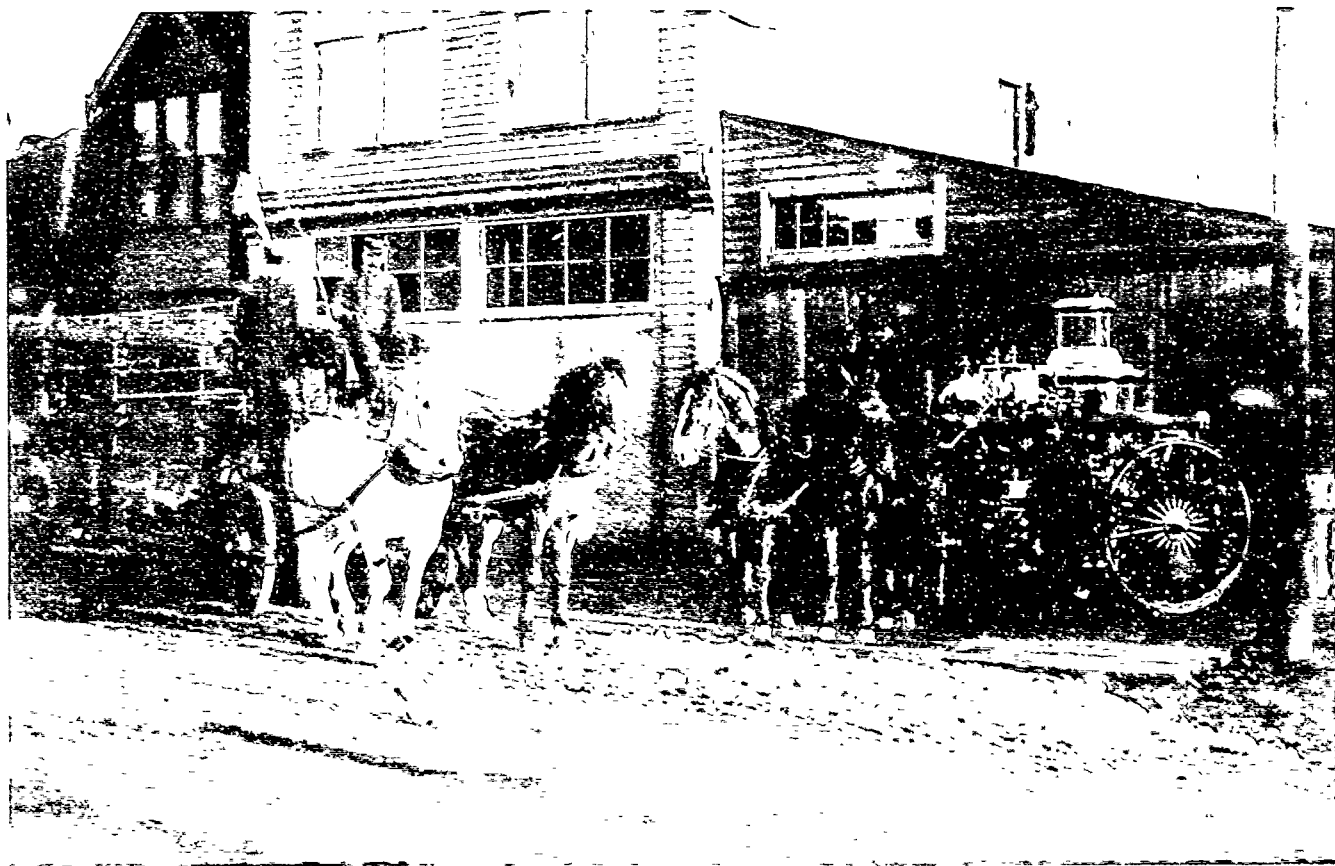
FIRE HALL NO. 2
