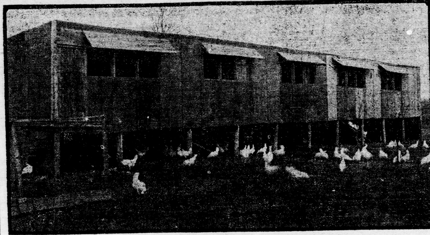
Part of the buildings on Mr. William Gurney's chicken farm on the Wharfedale road.
