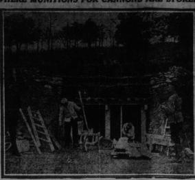
The above view shows a specially constructed shelter for storing shells behind the French lines. Two thick covering layers of earth are interposed between the magazine and the general level of the country around in order to lessen the risk of explosion should a chance shot strike the roof. The whole of this protective covering is carried on stout balks of timber and iron girders. The actual storage place is seen in the cavity behind the soldiers in the foreground.
