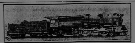
Introducing the M-1, just turned out by the Pennsylvania R. R. Altoona works, and said to be the engine in existence. It measures 84 feet 9 5-8 inches and weighs approximately 544,000 pounds.
