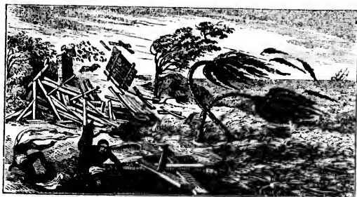
Hurricane in the West Indies.
