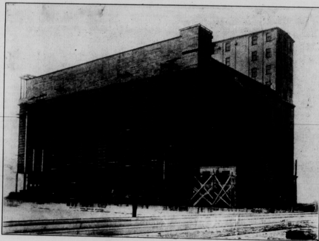
Dominion Government transfer elevator at Port Colborne, Ont. Extensive additions have been made to this house.
