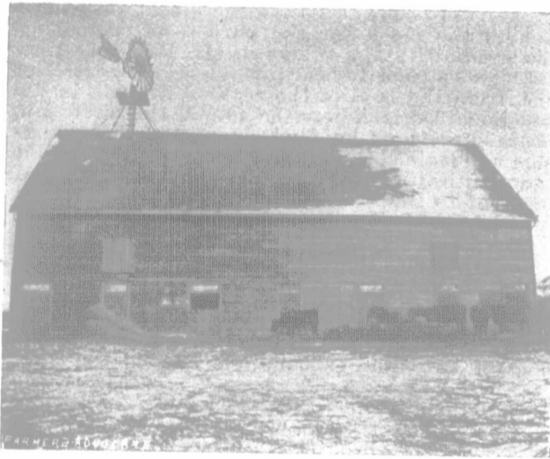
BARN—80X44 FT., CEMENT FLOOR—BUILT LAST YEAR BY JOHN G. BARRON, ON HIS FARM AT CARBERRY, MANITOBA.
