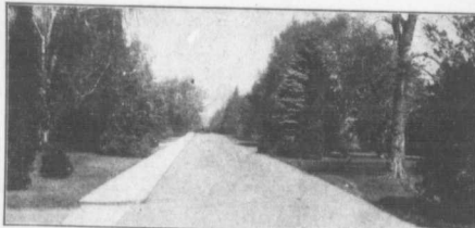
Driveway in Dominion Experimental Farm, Ottawa, Ont. Constructed with "Tarvia-X" in 1914.
