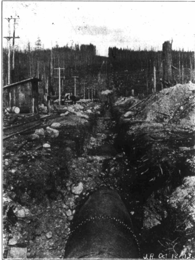
Fig. 10.— Pipe line right-of-way, showing No. 3 Pipe under construction.
