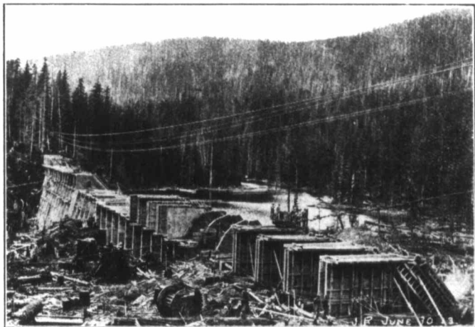
Fig. 5.—General view of the Jordan River Dam during construction.
