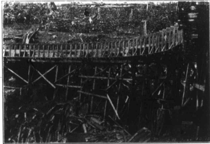
Fig. 8.—Jordan River Flume.—High trestle construction.
