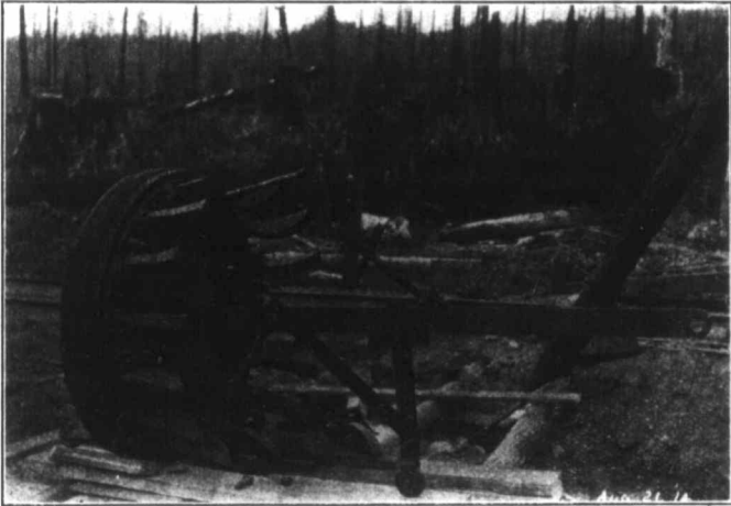
Fig. 11.—Bulkhead used for making tests on No. 3 Pipe Line.
