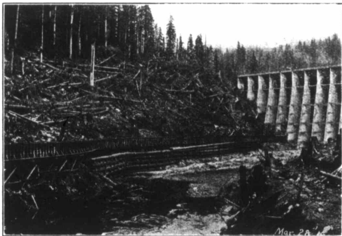
Fig. 6.—Crib work for protecting flume below Jordan River Dam.
