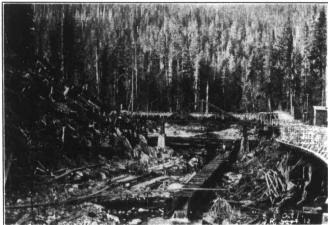
Fig. 2.—Starting construction of Jordan River Dam.
