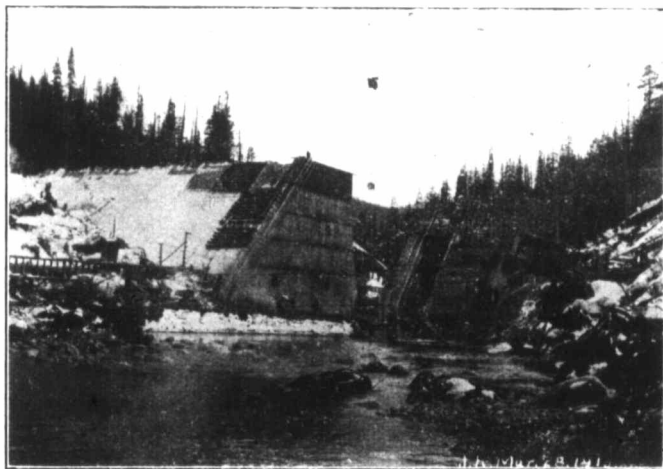
Fig. 4.—Looking down-stream, Jordan River Dam, during construction.
