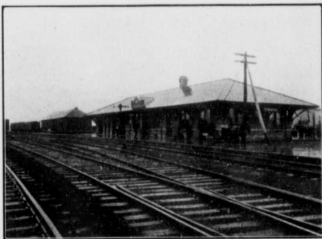
The T. & N. O. Railway station at Timmins.
