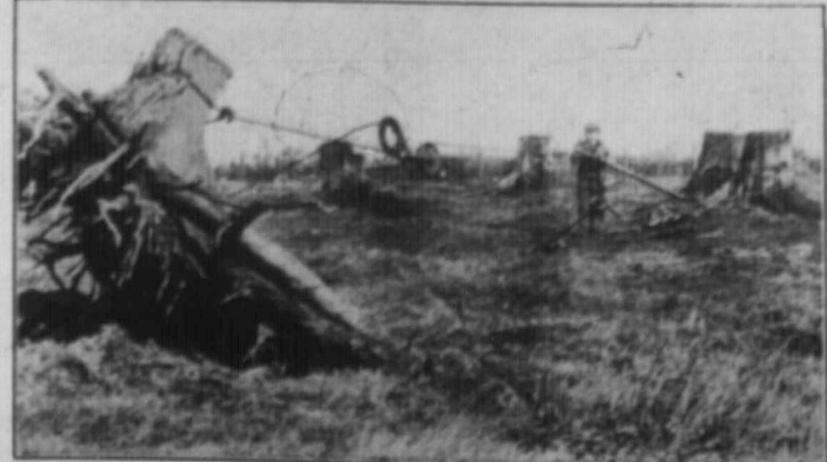
Uprooting a Big Fellow by means of a Hand-Operated Stump Puller
