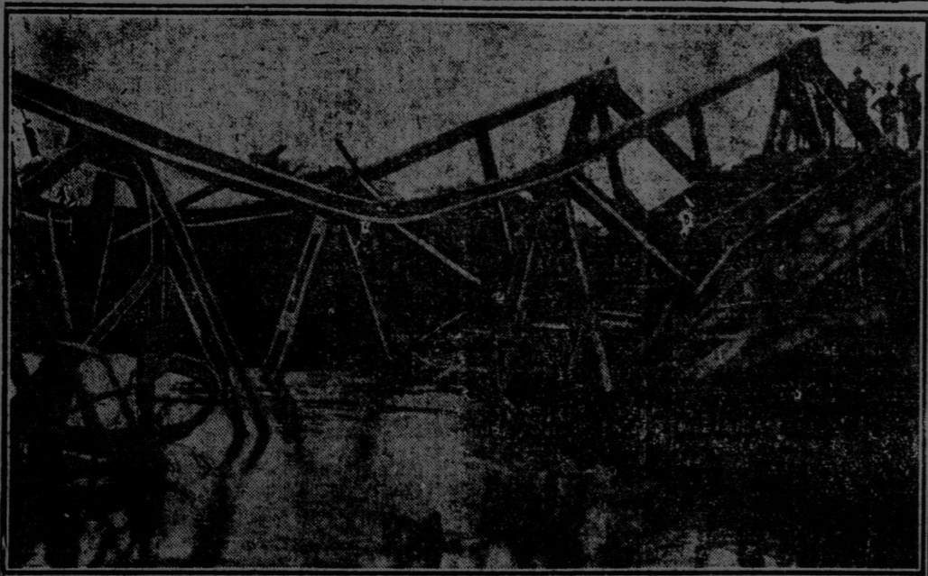
A railway bridge destroyed by Germans who were retreating in front of the successful British forces in the conquered German East Africa, which is now pretty well cleared of the foe. It will be noticed that the Germans have done their work of destruction pretty thoroughly, but in spite of this the British engineers had trains running over it again within two weeks.
