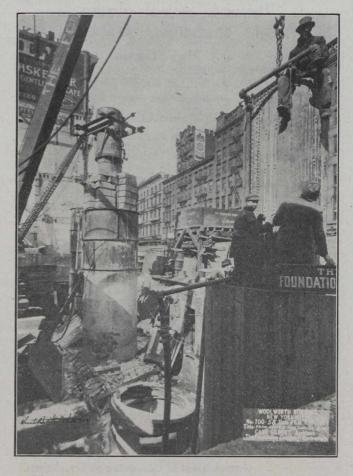
The site chosen for the building is unfortunately of a quicksand nature, and for this reason the foundation caissons have been t ken down no feet. This distance, with the height above the sidewalk gives the building a total elevation of 885 ft.
