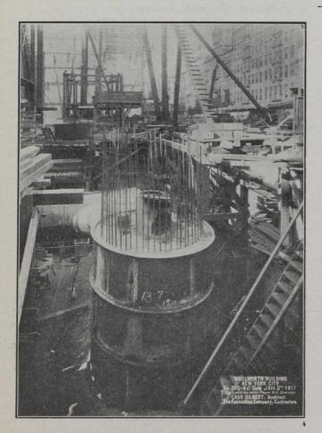
The four cuts are reproductions from photographs recently received of the site of the new Woolwarth building, New York City. Mention has been made from time to time in these columns regarding this structure, but these cuts of the foundations and the caissons used in their construction will not be out of place.
