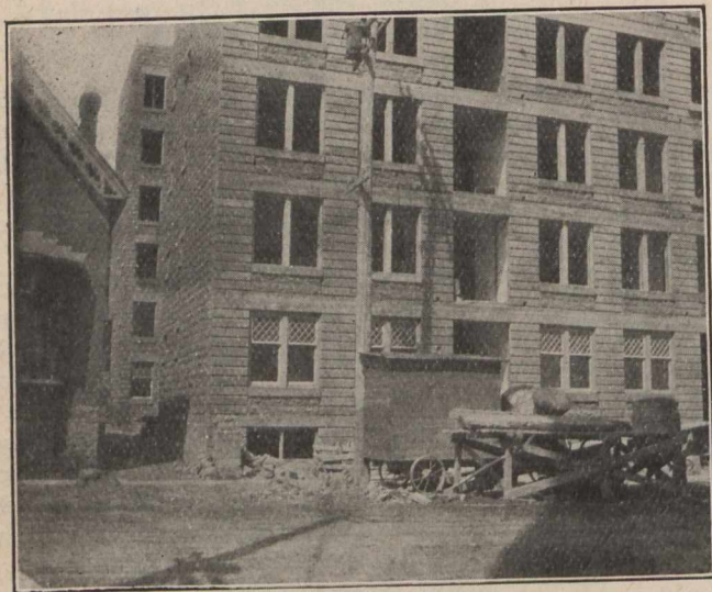
Apartment Block Under Construction at Ottawa.
