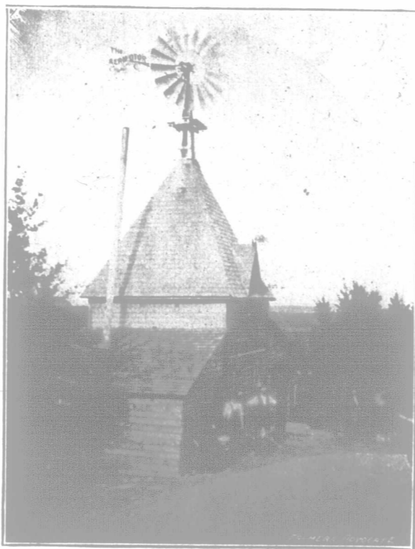
The Dairy Building.
