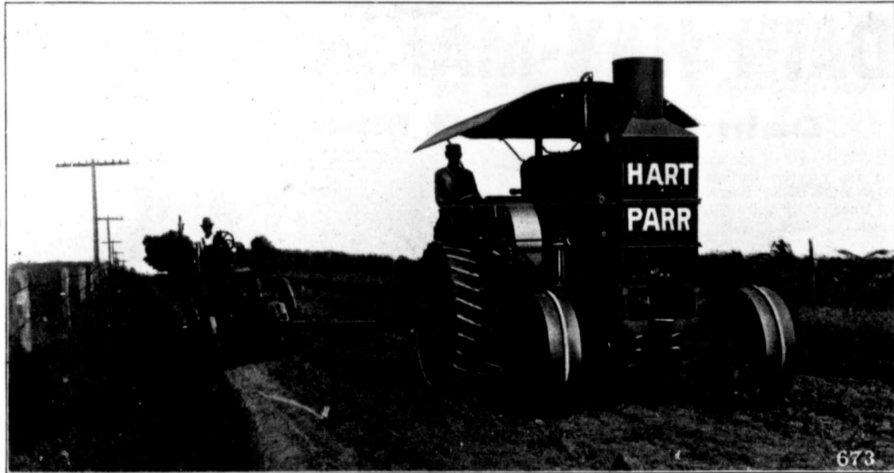
Shaping the Ditch with a Hart-Parr Oil Tractor and Blade Grader
