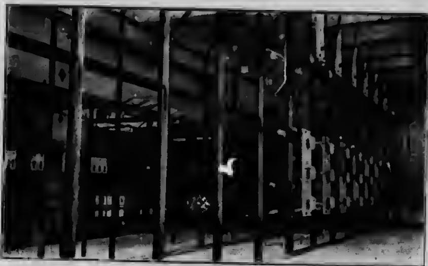
Olevano : High Tension Switches, (30,000 Volts).
