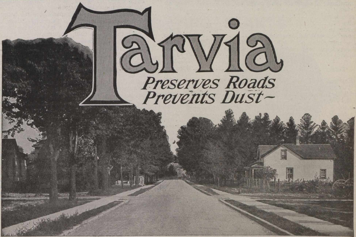
Charles Street, Stratford, Ontario, showing "Tarvia Modern Pavement."
