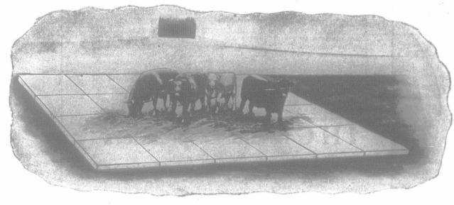
FEEDING FLOOR, 24x36 ft. -A feeding floor for sheep or cattle in the farmyard prevents loss and waste of hay, sait, grain, etc., and is easily cleaned. The illustration shows the general shape of a feeding floor which should be set an inch or two above the level of the farmyard, and also cast at a slight slope to allow water to run off.
