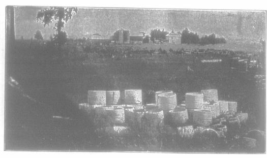
Fig. 10.—Cement tile after laying out on the surface over winter.
