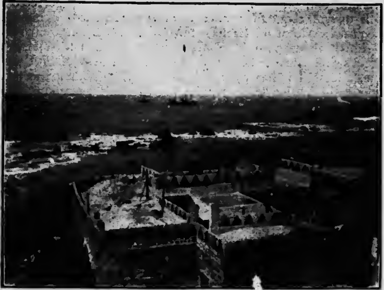
Joppa—looking from the roof of Simon's house
