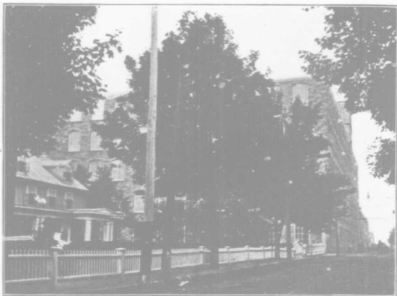
DUFFERIN ROAD, VALLEYFIELD, SHOWING EMPIRE MILL.
