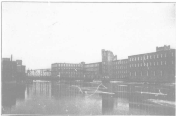
VIEW OF PART OF THE MILLS, FROM THE WEST
