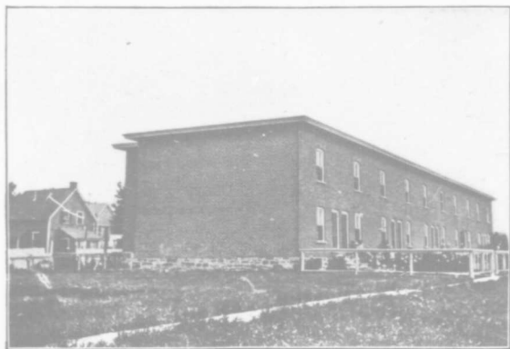
STEVENSON STREET, VALLEYFIELD
