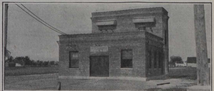
Chambly Sub Station.
