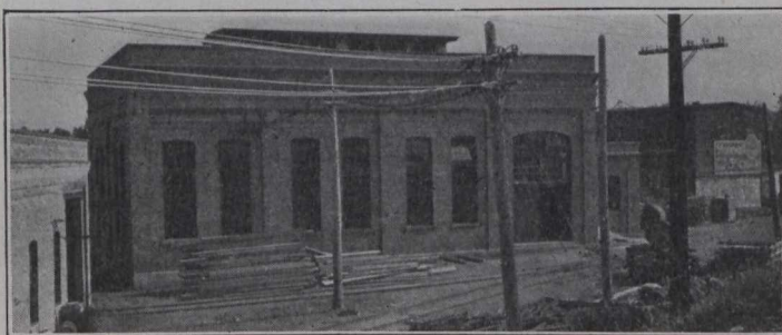
St. Lambert Sub Station.
