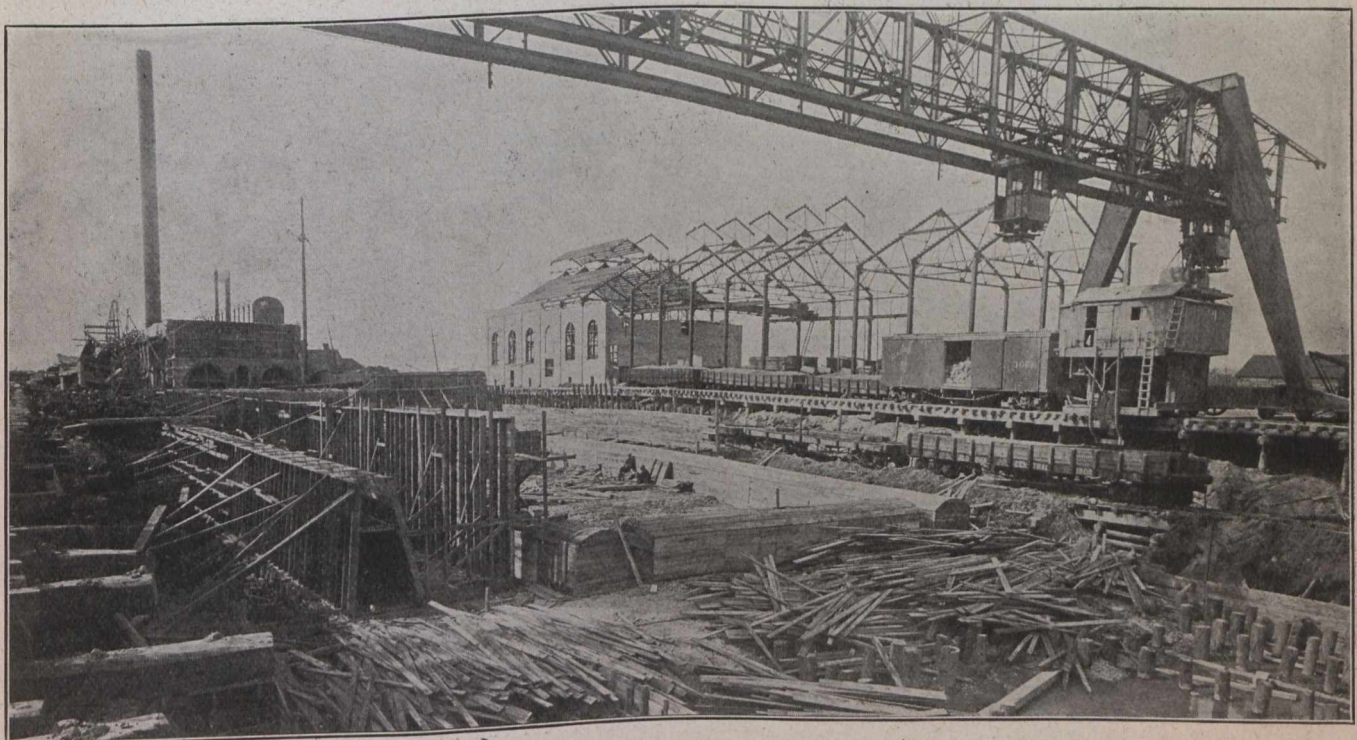
Fig. 6.—Progress Made up to October 6, 1910.
