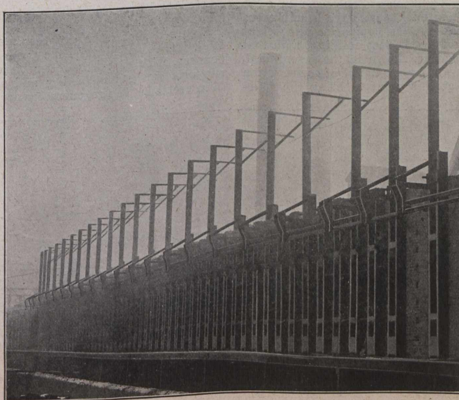
Fig. 10—Progress on Battery No. 2 up to March 1, 1911
