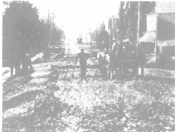
FIG. II.—ROADBED WITH FIRST LAYER OF BROKEN STONE, BEFORE BEING ROLLED.
