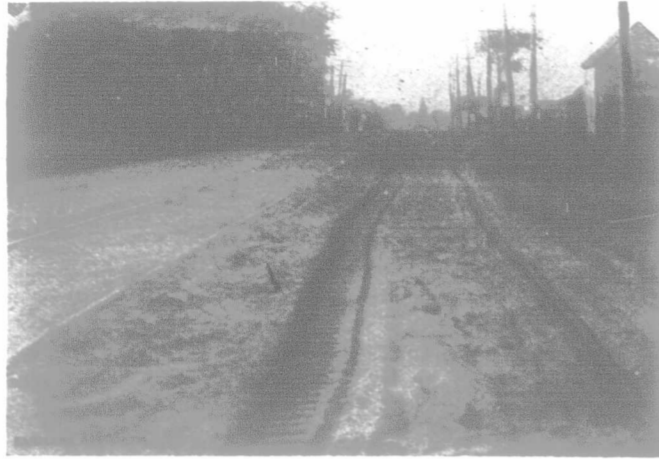
FIG. I.—SANDY STREET OVER WHICH THE MODEL ROAD WAS BUILT.
