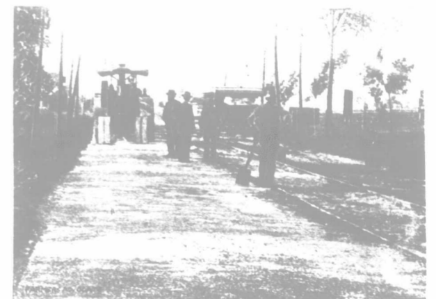
FIG. III.—PORTION OF ROAD ALMOST FINISHED.
