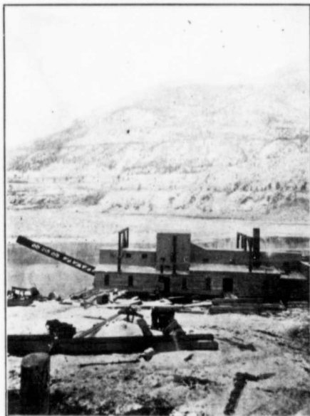
Dredge About Completed.
