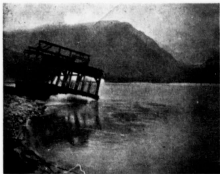
Dredge Being Launched.
