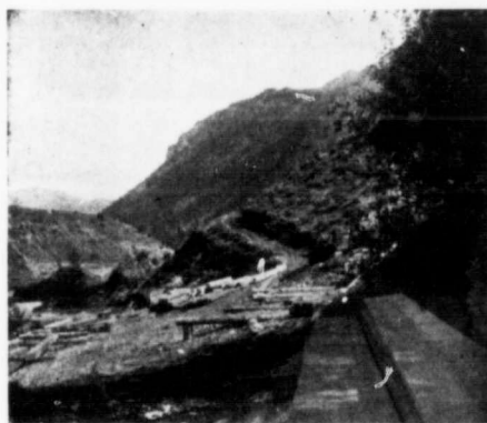
Road "from Lytton Road" to Dredge Site.
