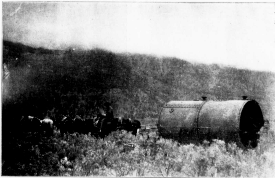
Boiler in Transportation.
