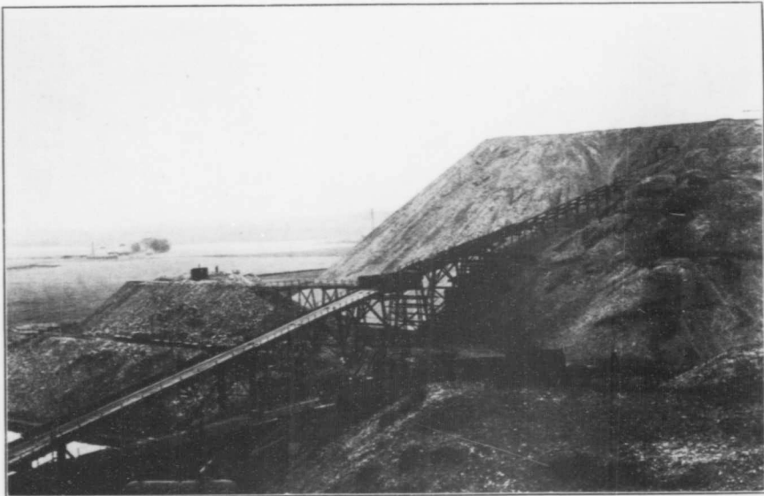
"Bings" or heaps of spent shale, with tramway from retorts to summit, Broxburn Works, Scotland.
