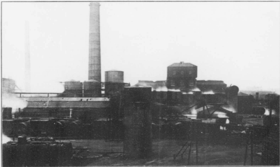
View in Refinery, Broxburn Oil Works.
