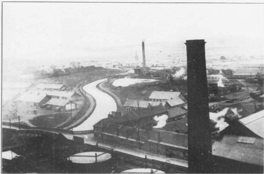
General view of Broxburn Refinery, showing the Paraffin House in the rear, and offices in front, Broxburn, Scotland.
