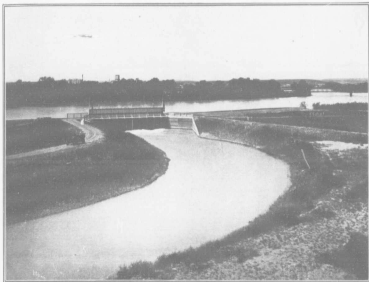
HEADGATES FOR MAIN CANAL C.P.R. IRRIGATION SYSTEM, EAST CALGARY
