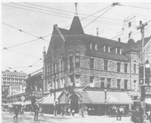
CORNER OF EIGHTH AVENUE AND FIRST STREET WEST
