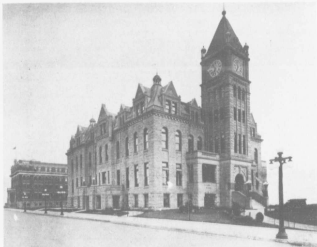
CITY HALL, CALGARY, SHOWING POLICE BUILDING ON SEVENTH AVENUE
