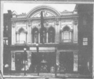
FRONT OF ALLEN THEATRE CALGARY THIS IS THE FIRST LARGE THEATRE CONSTRUCTED BY ALLENS. NOW THERE ARE MORE THAN 60 ALLEN THEATRES IN CANADA.
