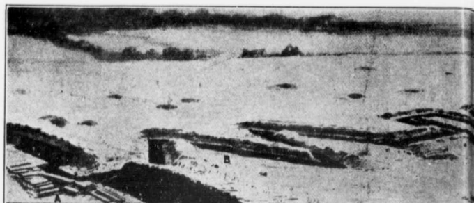
MINING. TRENCH AND SAP - A PERSPECTIVE VIEW - AFTER OPERATION
