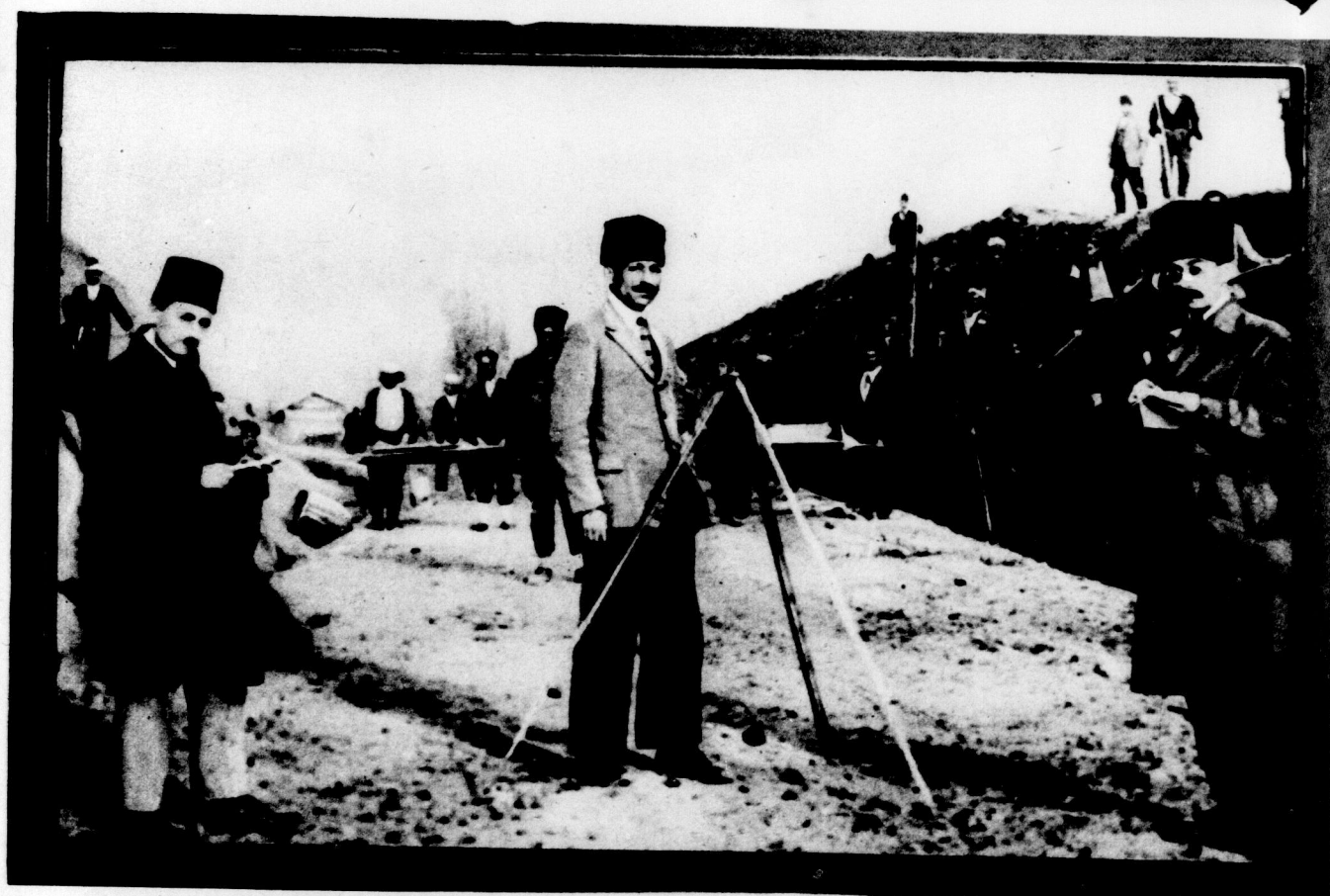
Beginning construction on the Samsoun-Sivas railway in Turkey, which will open up the vast wealth obtained by British and United States interests through the famous Chester concessions
