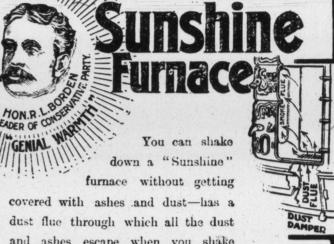
and ashes escape when you shake down the fire. This heater is so easily regulated and operated,
