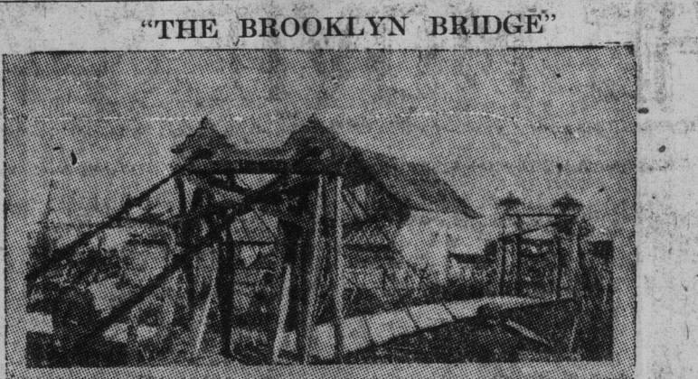
Not across the East River, but soon elsewhere in France. Temporary structures such as this bear much important traffic behind the front.
