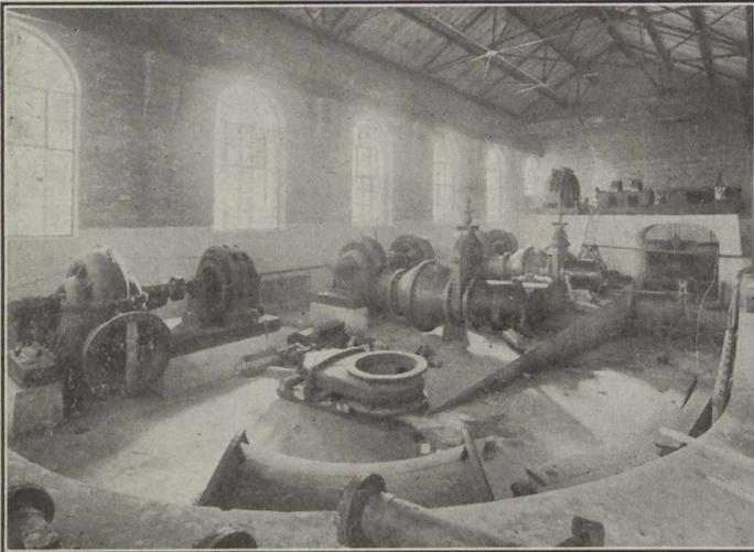
Fig. 6.—Southern Part of Pumping Station, Showing the Three Pumps with Direct-connected Motors and Generating Unit in Background.
