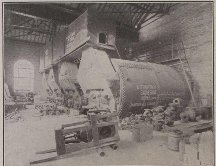
Fig. 5.—Installation of Boilers in Progress.
