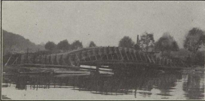
Fig. 7.—Falsework and Forms During Concreting.
