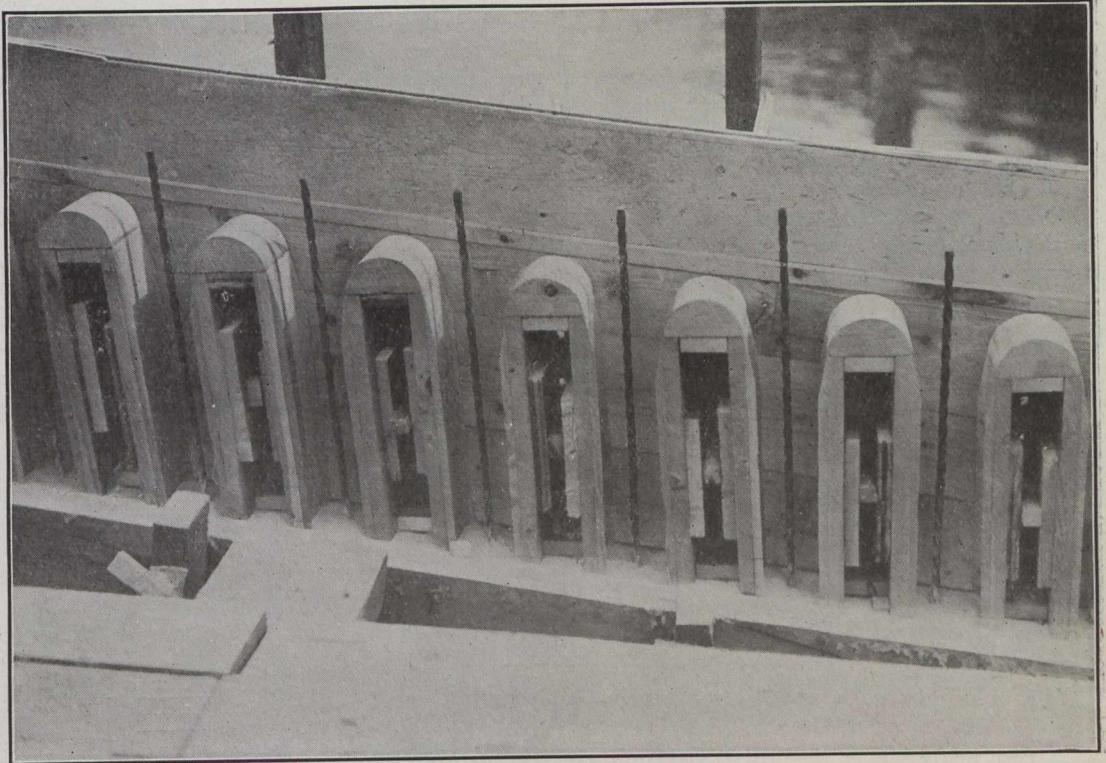
The order in which the concrete was placed is as follows: First, the abutments up to the springing; second, the arch rib working from both ends at the same time in order to produce symmetrical deformations in the falsework; third, the parapet walls; fourth, the spindles and railing.
