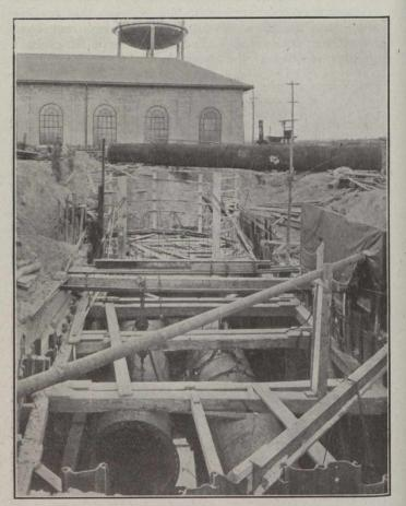
Fig. 8.—View of Intake Pipe Trench at North End, Showing Commencement of Laying Two Lines of 72-inch Steel Pipes.
