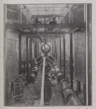
Fig. 3.—Filter House During Installation of Pipe Connections in Central Gallery. View Looking North.
