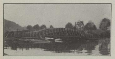
Fig. 7.—Falsework and Forms During Concreting.
