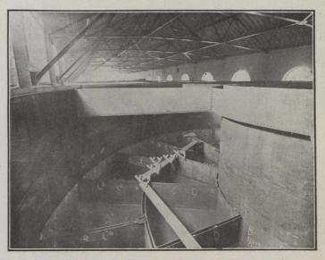
Fig. 4.—Interior View of Section of Filter Tank.
