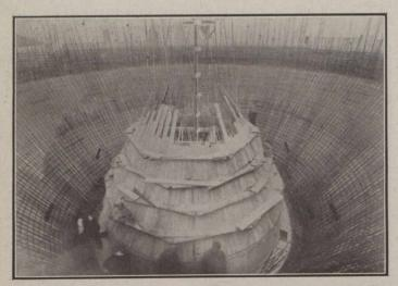
Fig. 7.—Interior View of Chemical House, Showing Reinforcing in the Bottom of the Cone-shaped Storage Bins for Alum.
