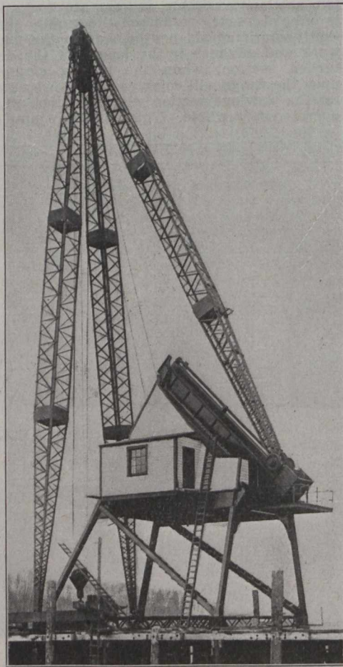
Pier Derrick at Grand Trunk Pacific Railway's Ship Repairing Plant, Prince Rupert, B.C., Capacity, 50 Tons.
