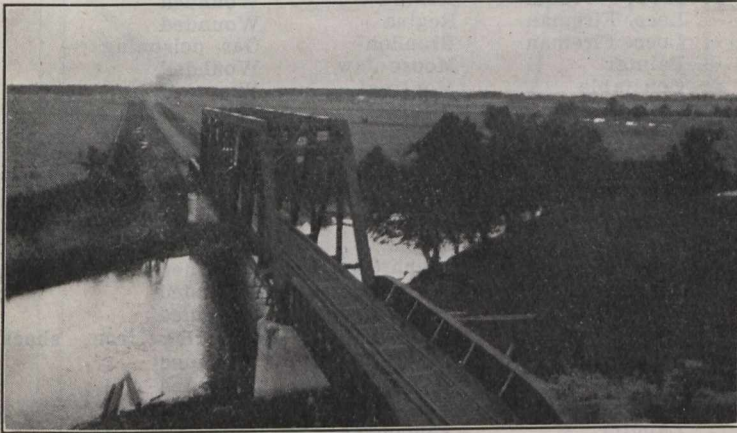
Carp River Bridge.
