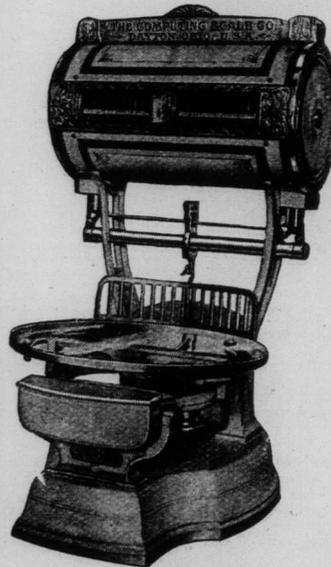
All that is necessary to get the value of a piece of merchandise at any price per pound shown on the chart, and at any weight up to and including the full capacity of the scale is to put the merchandise on the platform of the scale.
