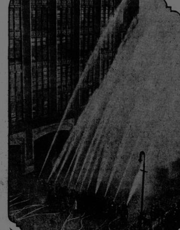
Boston Fire Department tested out the new high pressure system by playing 12 high-pressure streams into Boston harbor. Note the height attained. The test was satisfactory.
