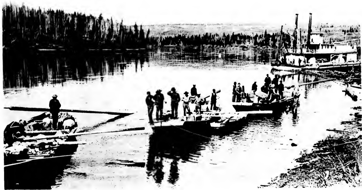
BOATS WITH FREIGHT LEAVING THE LANDING FOR THE FAR NORTH.
