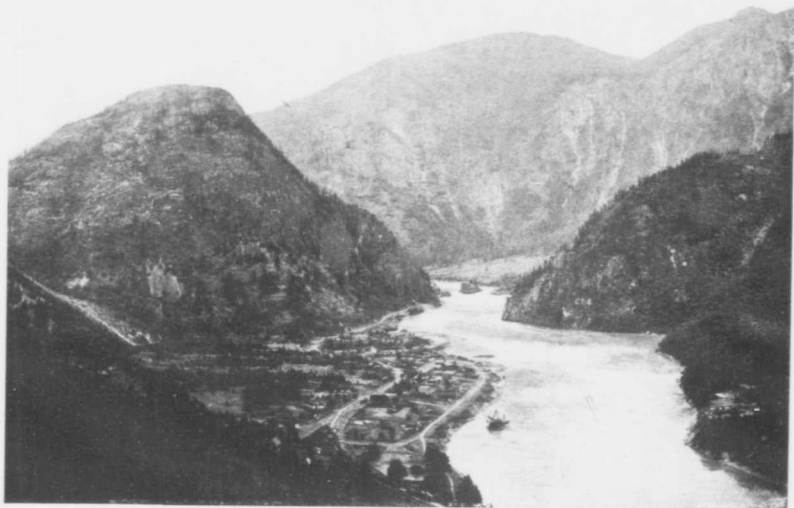
YALE, B.C., AT ENTRANCE TO FRASER CAÑON.
