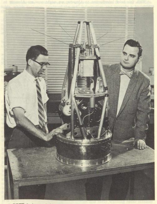
DRTE instrumented a Javelin rocket nose cone which was fired in the U.S. to prove the efficiency of the Alouette antennae system. This is a prototype of the nose cone with some of the DRTE instrumentation employed.
