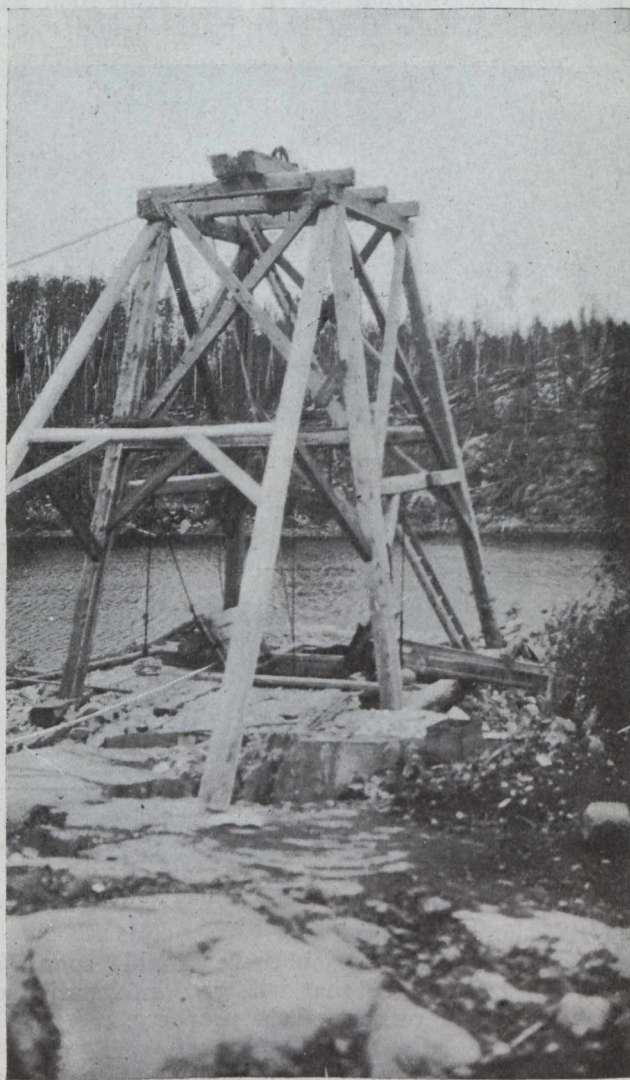
The West Tree Headframe.
