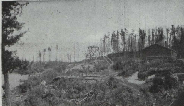
A View of the West Tree Headframe and Power House from the North.
