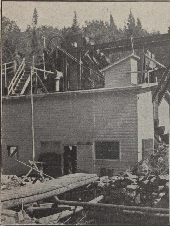
Hydraulic Plant at Beauce
