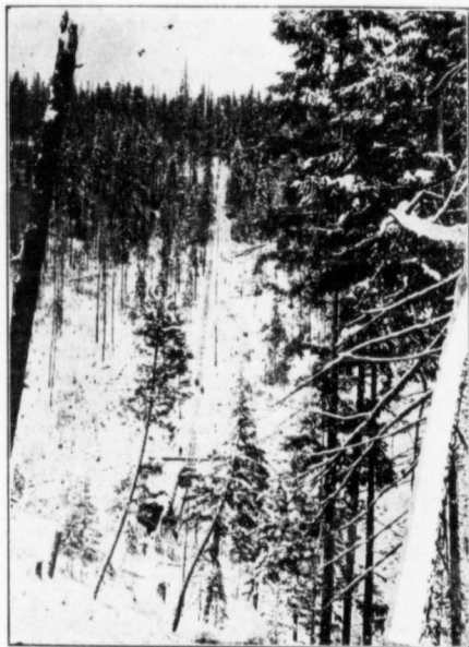
E. P. U. Mines Gravity Tramway, near Greenwood.
