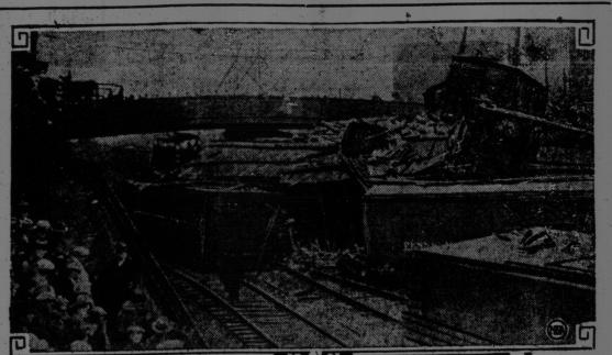
A long string of freight cars on the Pennsylvania railroad got loose on the famous "horse shoe curve" near Altoona, Pa., and reced down a steep two-mile grade into the city. There the cars side-swiped" another string and were wrecked, blocking all traffic on the main line and killing two trainmen. The brakeman saved his life by running back along the tops of the cars. There are 19 cars piled up in the heap
