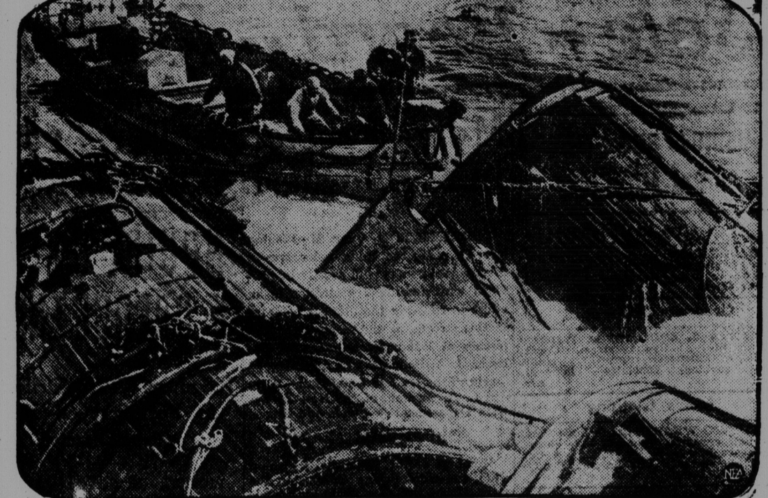
GIANT pontoons had just raised the nose of the lost Navy submarine S-51 above the waters off Block Island, R. I., when—crack!—a cable snapped. Months of work by a gallant salvage corps went by the board as the heavy ship sank back to the ocean bed. The nose of the submarine can be seen in the centre of the picture, supported by pontoons, an instant before the mishap.
