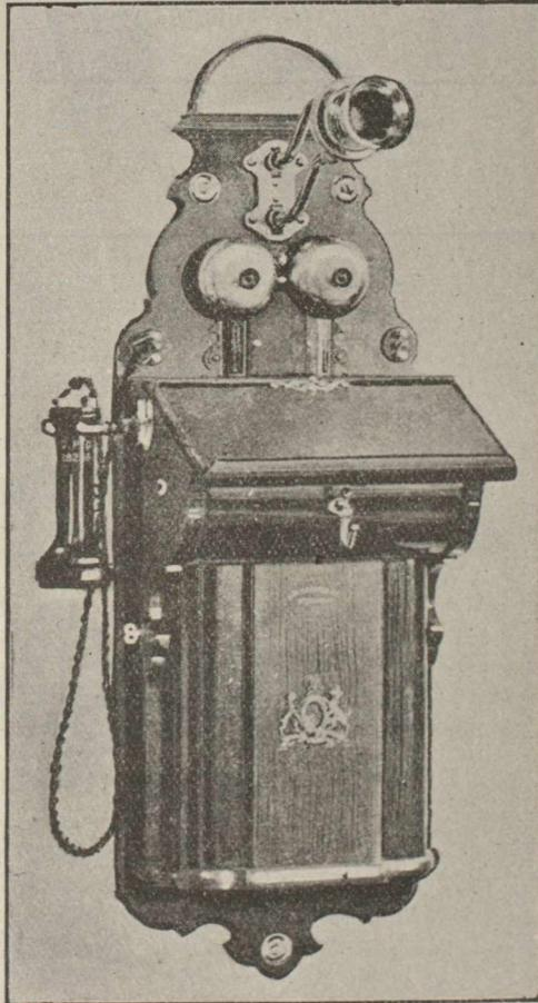
FIG. 4.—WALL TELEPHONE FOR SUBURBAN EXCHANGES
